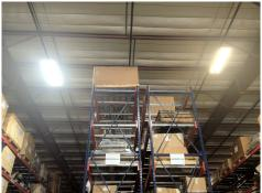
Image to the right shows on the left Orion's 4-lamp T8(145 watts) full power and the competitor's 4-lamp T5(214 watts) fixture on right. Orion fixture is putting out 18.3 foot candles and competitor fixture is putting out 13 foot candles.
