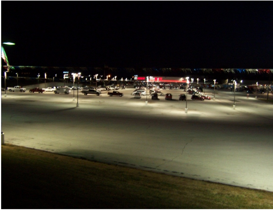
Pre-Installation – Approximately 28 Foot-candles
